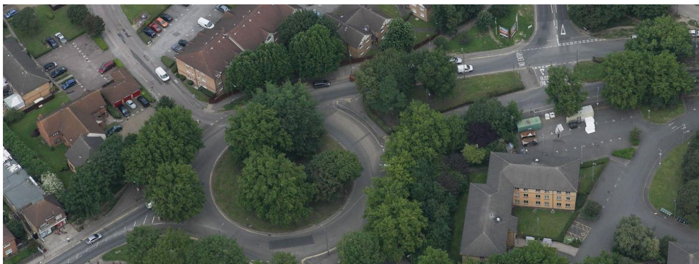
» Current Colindale Roundabout aerial view
