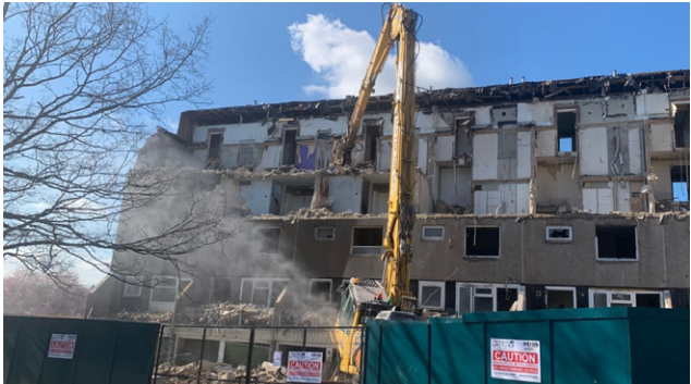
» Demolition of 1-42 Garrowsfield residential block
