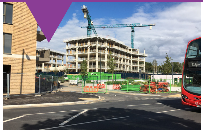
» Millbrook Plaza under construction
