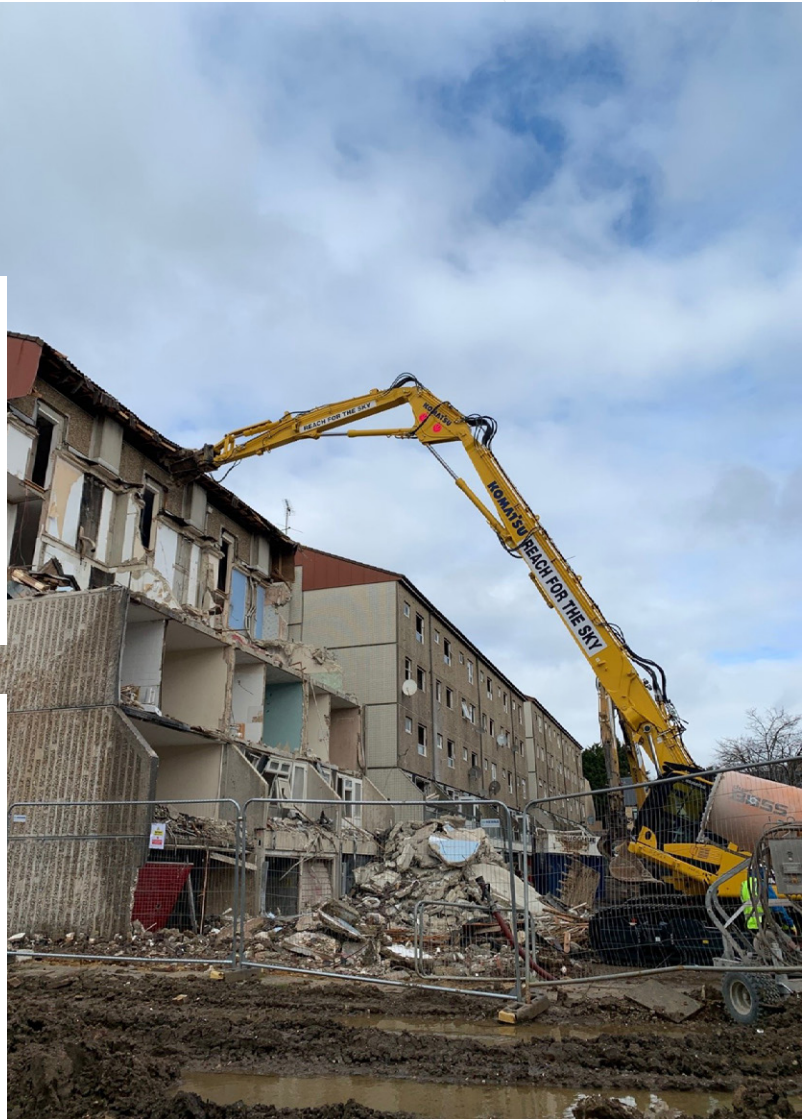
» Demolition of 90-124 The Ridge residential block
