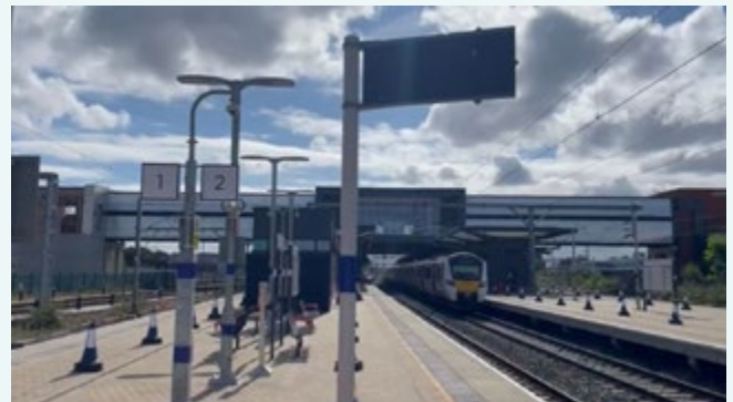
Brent Cross West station platform
