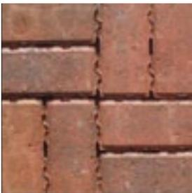
**Brick Pavers:** The most traditional style of permeable paving. Water is allowed to penetrate into the ground through the gaps between each paver. It is important they are laid correctly onto a compacted aggregate so the water can drain away freely, and the correct depth of sand (no more than 30mm after compaction.)
