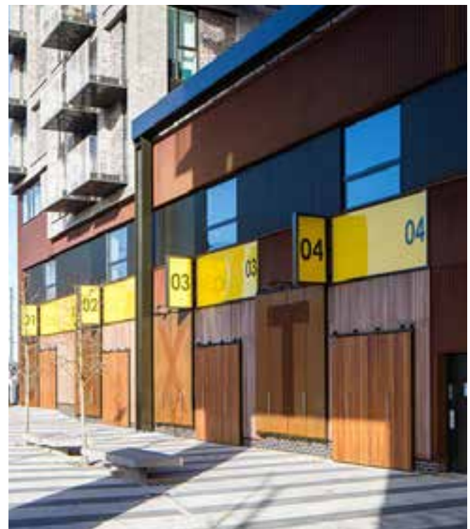
Caxton Works_ External View
