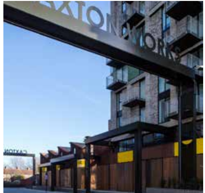
Caxton Works_ External View
