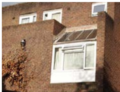
Existing 3 storey townhouse type on site, with 'winter garden' at the rear
