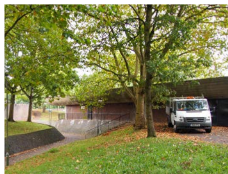
Existing energy centre
