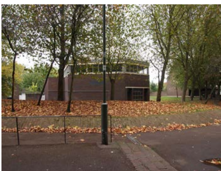
The existing church
