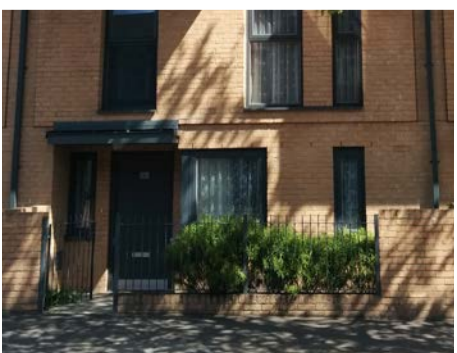
Defined front gardens with permeable frontage for planting, Hammond Court, Waltham Forest
