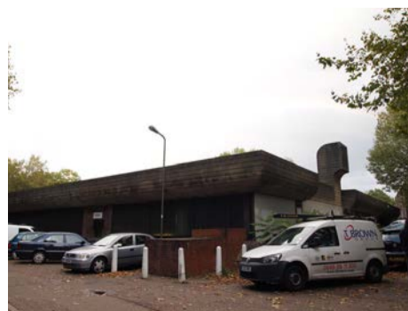
Existing energy centre
