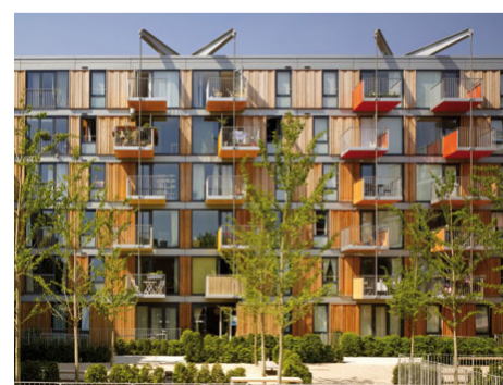
Prominent, lively frontage, Adelaide Wharf, Haggerston
