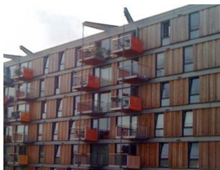
Prominent, lively frontage, Adelaide Wharf, Haggerston
