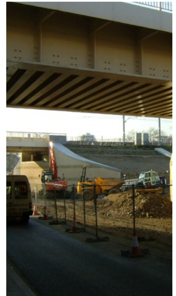
The new Aerodrome Road bridges being constructed
