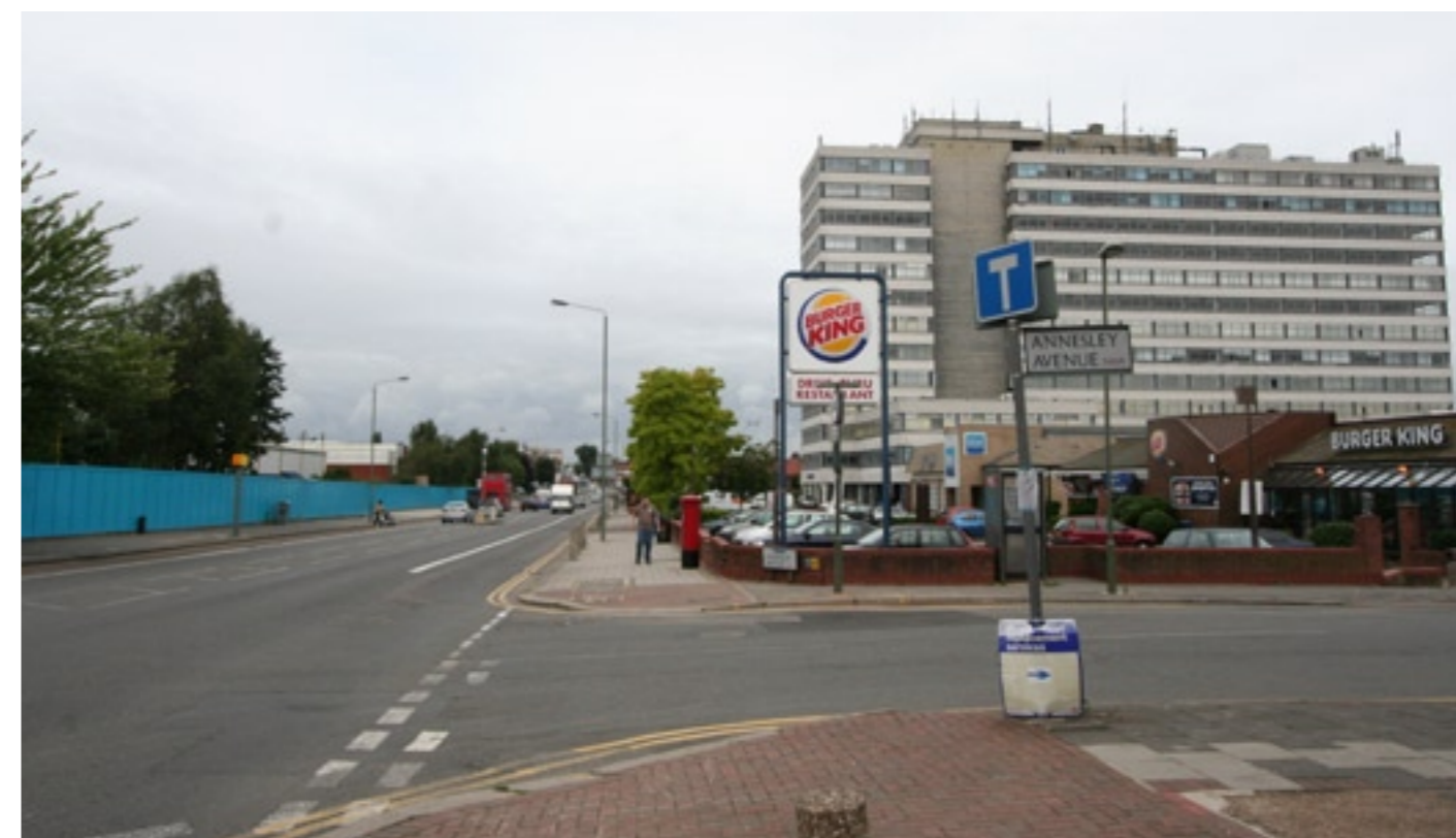
Burger King/D&A site, Merit House (tall office building) looking west along Edgware Road
