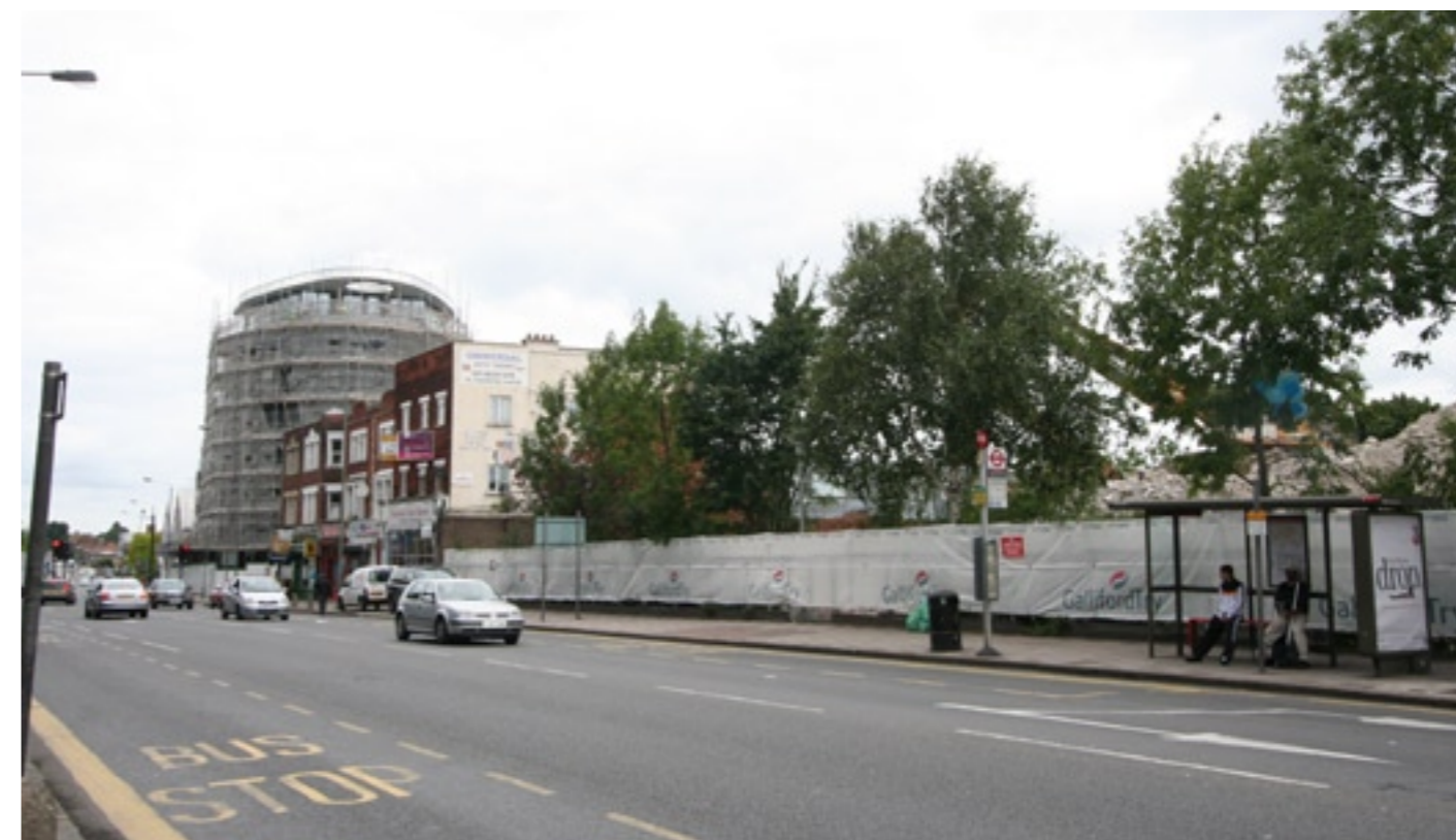
Zenith House site (to the right), former Kidstop site (under construction) and junction of A5/Colindale Avenue looking west along Edgware Road
