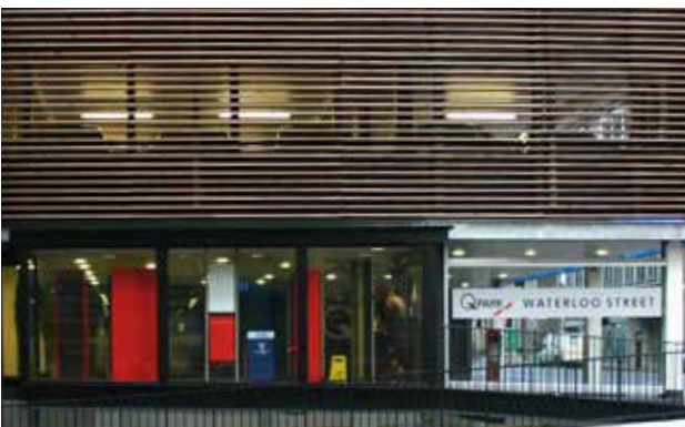
Image 34: Decked car park with active frontages
