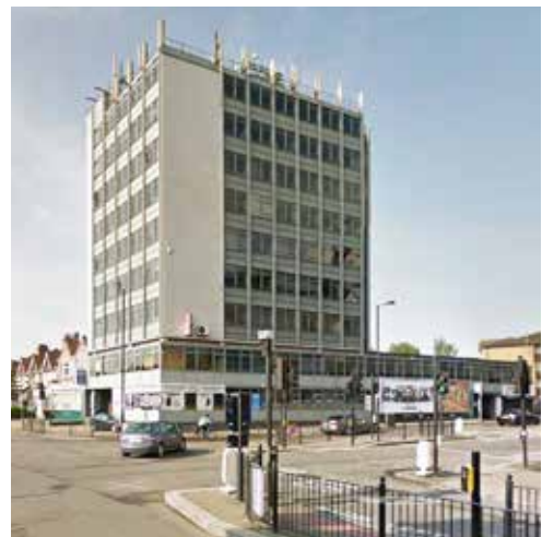
Image 15: street view of existing office building
