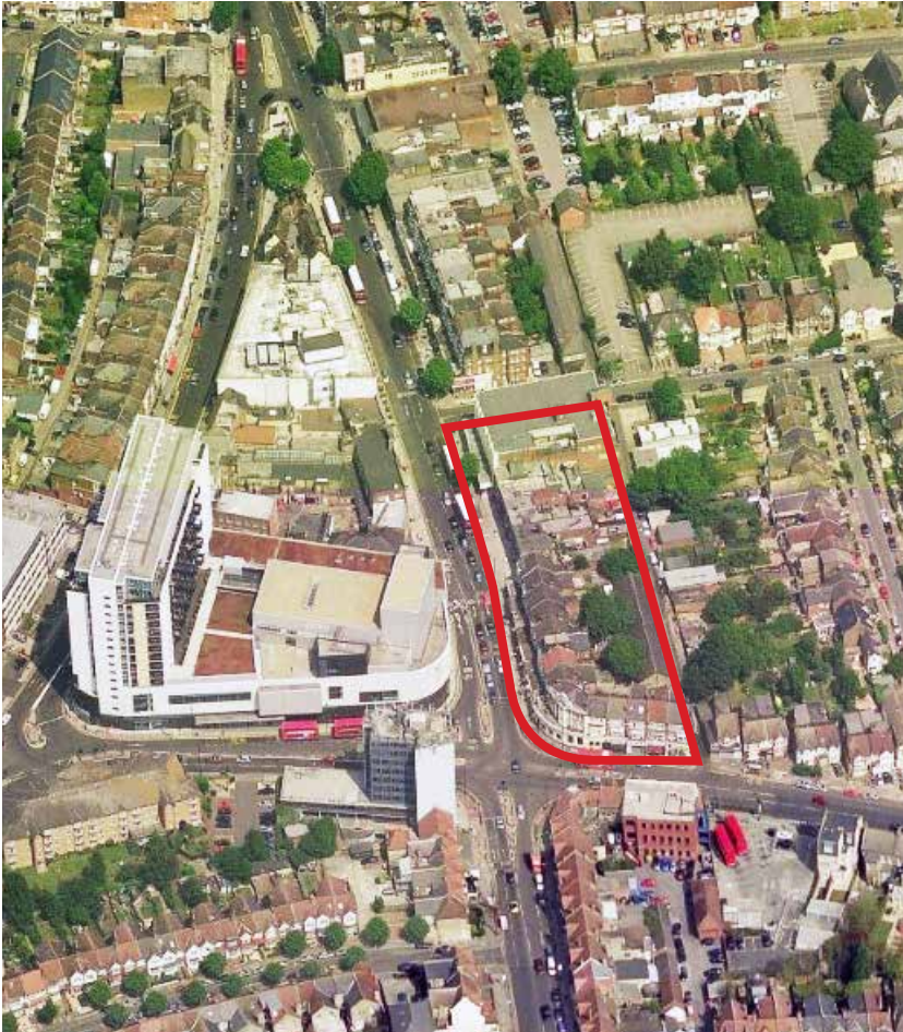
Image 20: existing aerial view of East Wing site
