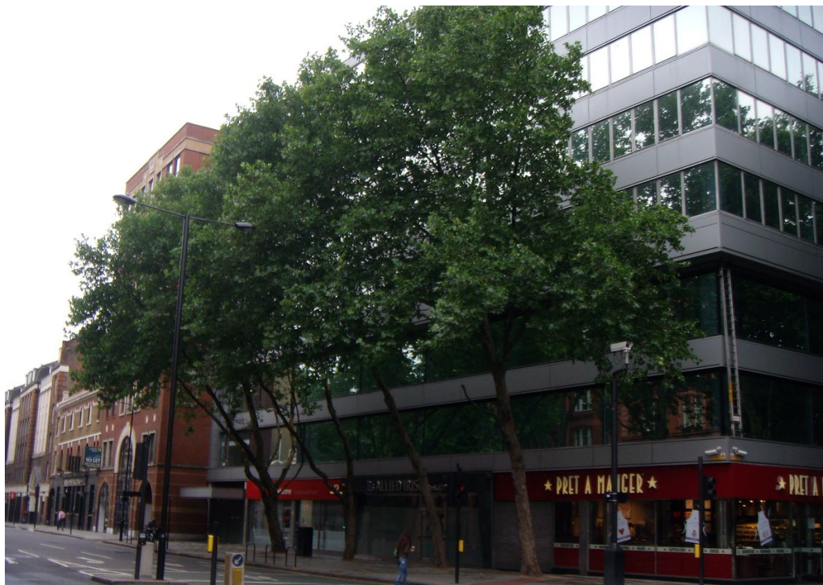
Figure 14 - Copse of trees planted to mitigate windy conditions near building corners
